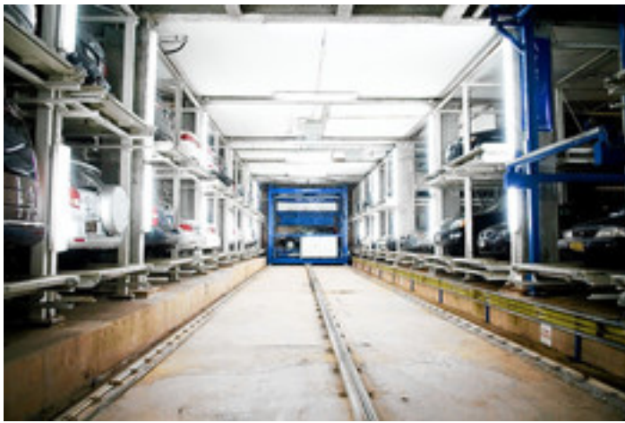
Rob Bennett for The Wall Street Journal A conveyor belt moves a car on its pallet to a snug, automated parking slot at the garage on Baxter Street.
